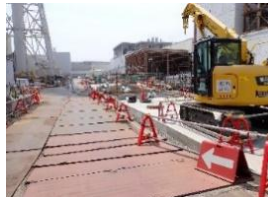
Before facing (near Unit 3)
