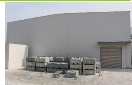
Exterior view of solid waste storage 10 (Source: TEPCO)
