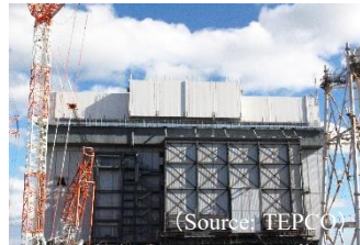
Installation of a large cover for Unit 1 was completed.
