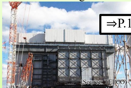
TEPCO's Fukushima Daiichi NPS Unit 1
