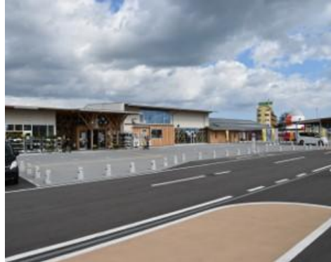
Namie Town: Roadside-Station "Namie"
