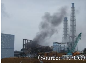
Unit 3 immediately after the hydrogen explosion
