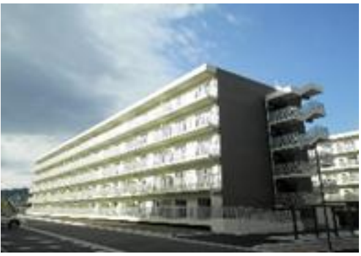
Minamisoma City: Minamimachi Housing Complex
