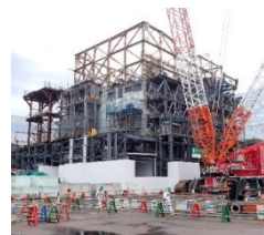
Installing a large cover for Unit 1
