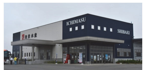
View of the reconstructed Shibaei Suisan
