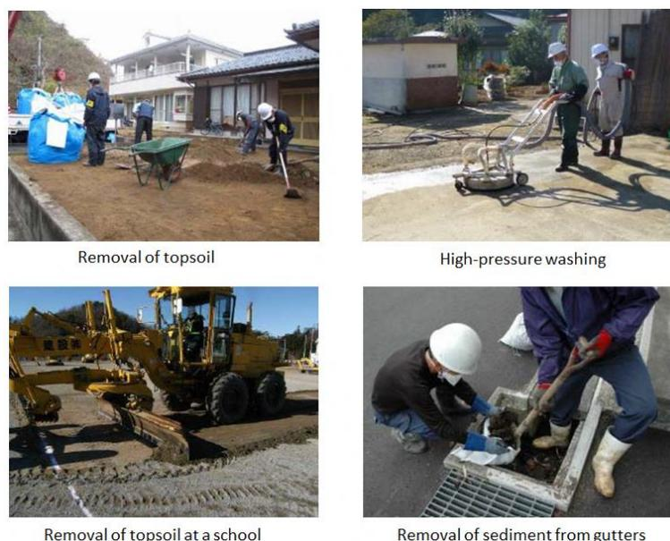
FIG. 3.13. Main decontamination techniques (Image: Fukushima Prefecture)
