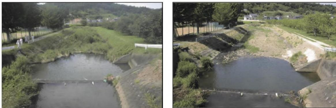
FIG 3.9. River bed before (left) and after (right) decontamination measures in the Kami-Oguni river (Image: Fukushima Prefecture – presented in ‘previous report’).
