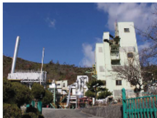
※CFT(Coal Firing Test Furnace)
