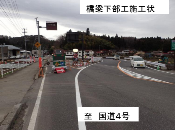
橋梁下部施工工状
